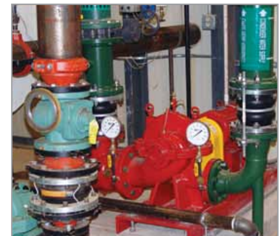
Highly Efficient, Green Installation
