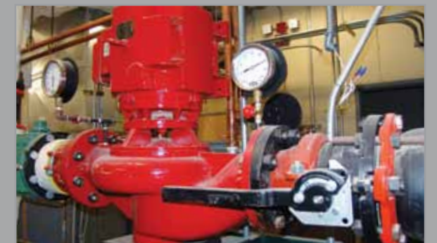
Woolworth Building —EnviroFlo Close-Coupled Vertical In-Line Pumps are providing world-class quality and reliability as they circulate condenser water to 18 units on three floors of this world-renowned structure in NYC.
