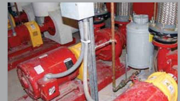
Rhode Island School of Design—EnviroFlo Frame-Mounted End Suction and Vertical In-Line Pumps are maintaining critical climate control requirements in a 128-year-old library while minimizing energy consumption.
